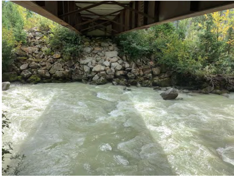
Left Bank Abutment when facing downstream
