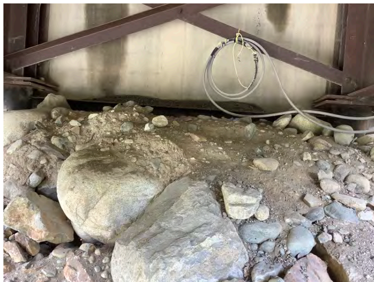
Right Bank Abutment when facing downstream
