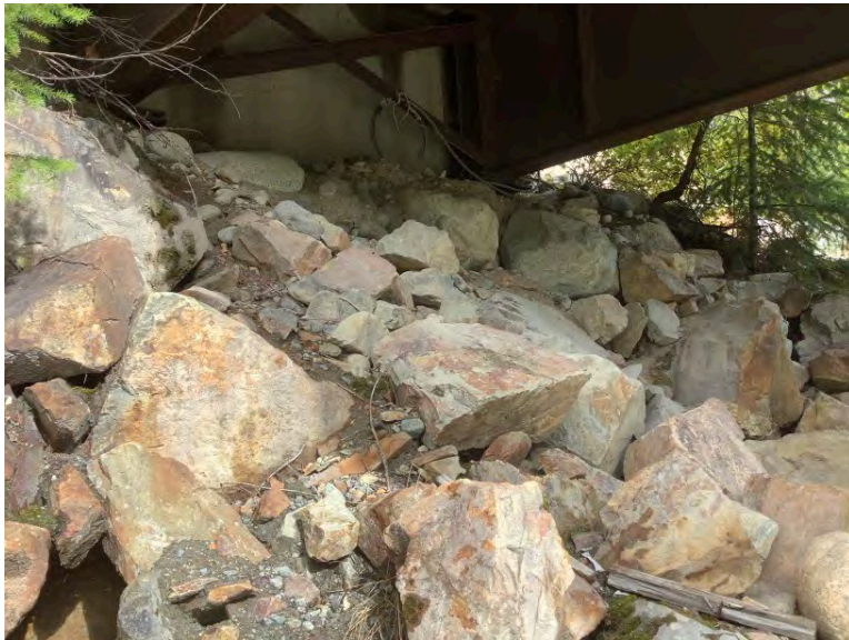
Right Bank Abutment when facing downstream
